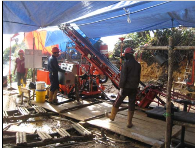
Figure 27: PT Antero Indodrill AD200 Drill Rig (ID-350D)
